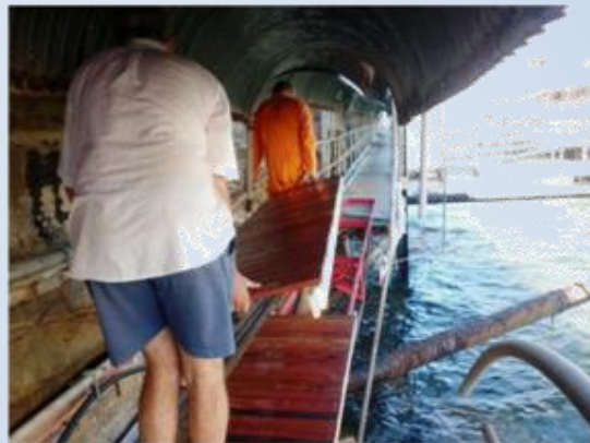
Laying the bridge top
