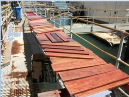
Planking the bridge
